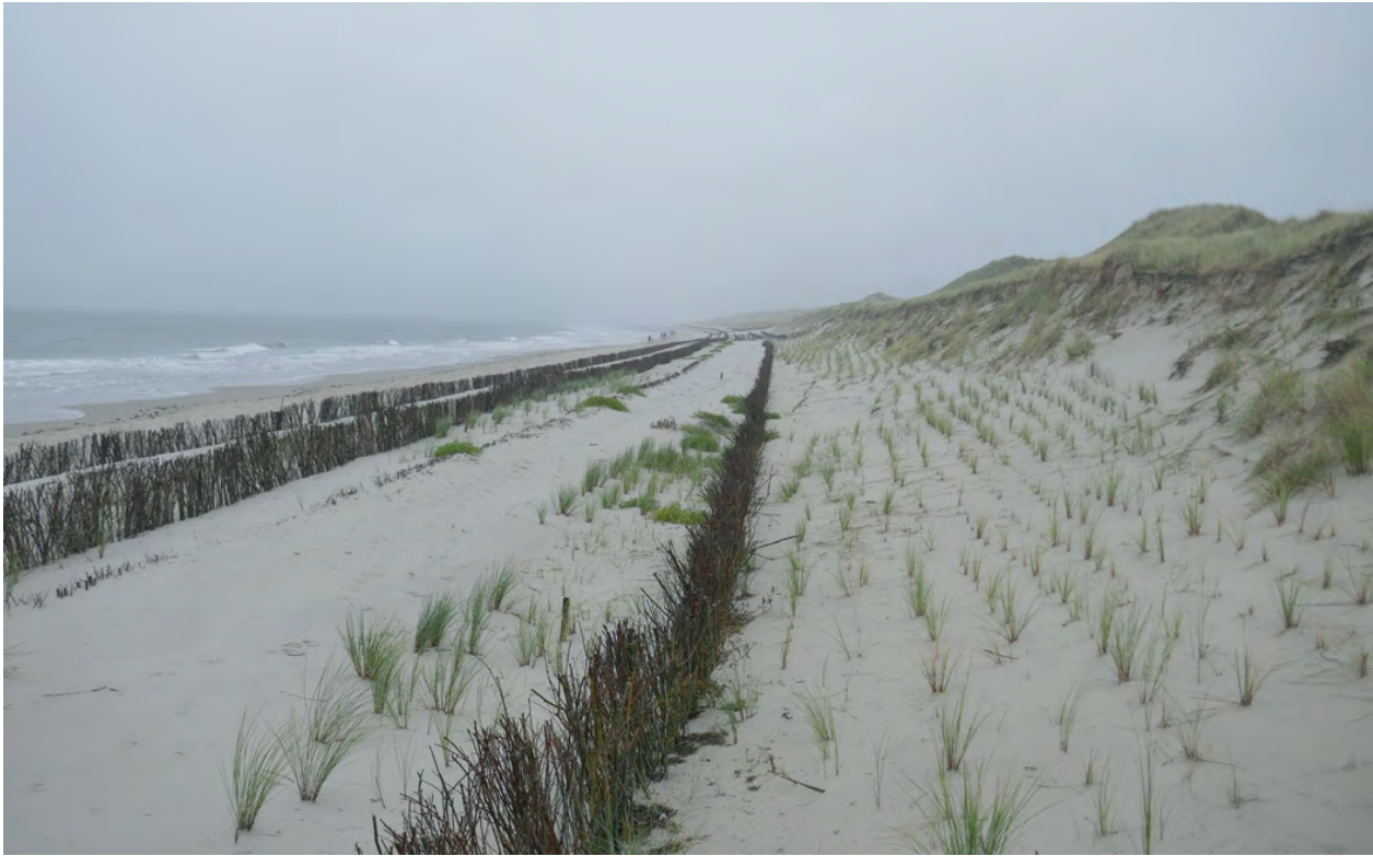
Figure 5.8: Amrum, Germany: Fresh stalk plantings and sand trapping fences to secure and further build up the coastal dunes that protect the island of Amrum, Germany. Photo: Philipp Jordan.
